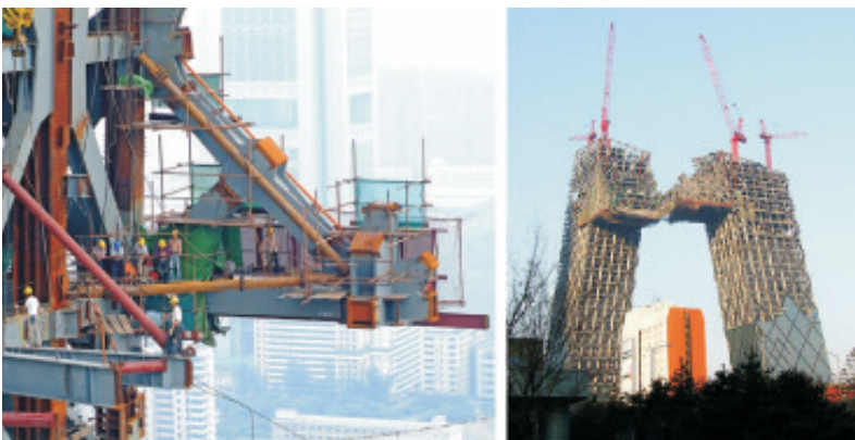
Figure 11: Cantilevering the top bridge structure (source: Ref. 12)
