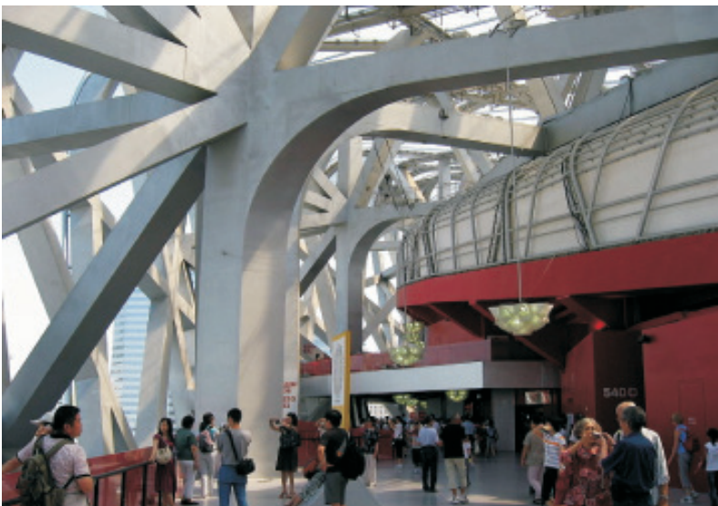
Figure 3: Interior view of Bird's nest stadium showing the interior main columns, truss members, secondary and tertiary steel members and their connections (Source: http://en.wikipedia.org/wiki/Beijing_National_Stadium )
