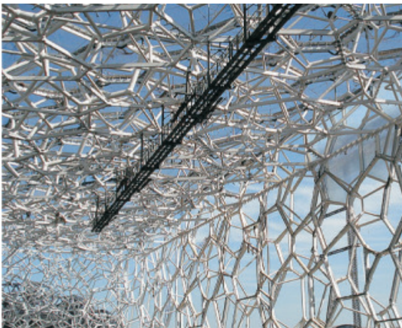
Figure 6: Steel superstructure of the National Aquatics Centre (source: http://www.arupinbeijing.com/arup_projects/national_aquatics_center/ )
