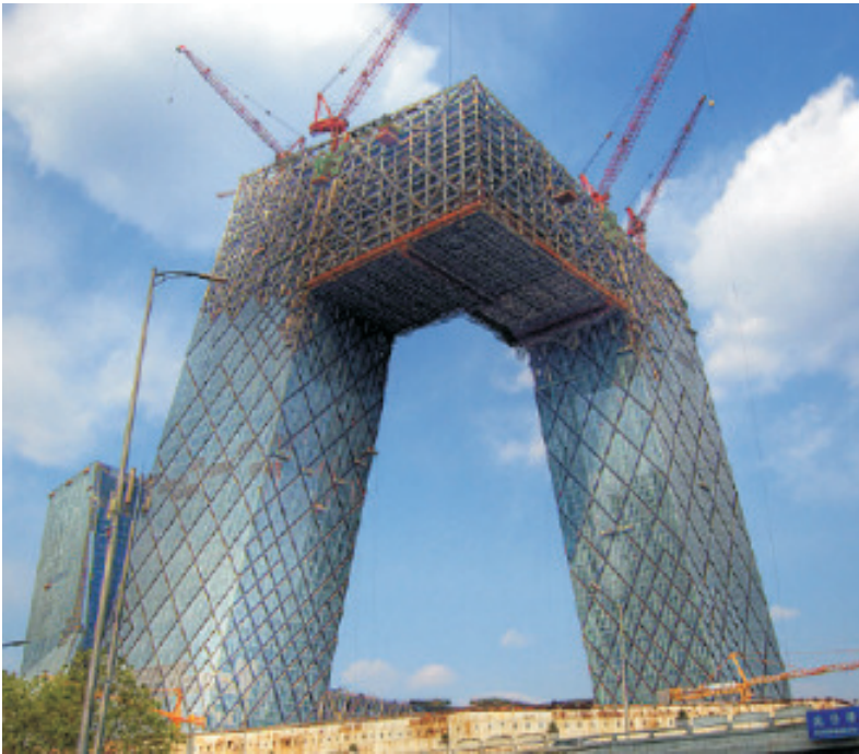
Figure 9: View of CCTV Tower under construction (Source: http://en.wikipedia.org/wiki/Image:CCTV_Beijing_April_2008.jpg )
