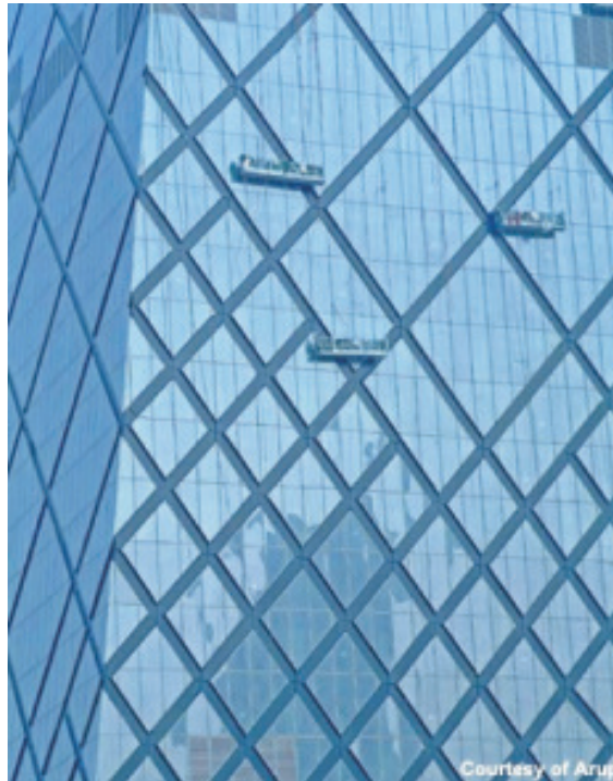
Figure 11: The external skin of the CCTV building has a diagrid exoskeleton which makes the tower act as an integral tubular unit (Source: Ref.11)
