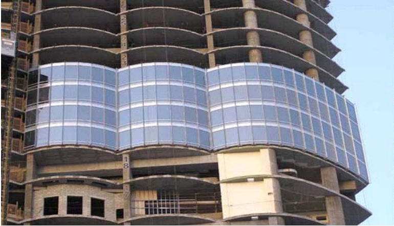
Fig. 8 High performance exterior cladding system was used to withstand the extreme temperatures during the summer months in Dubai (Source: Ref. 5)
