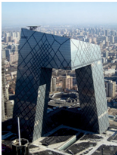
The CCTV Headquarters, Beijing
