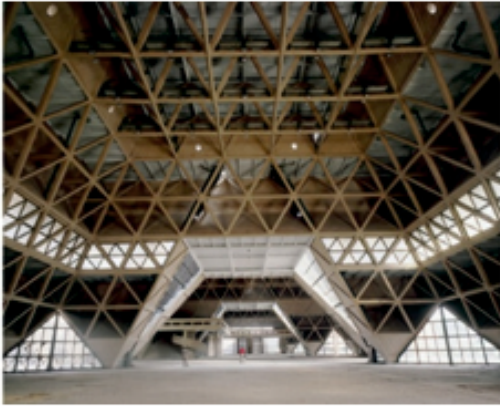
The Hall of Nations at Pragati Maidan, Delhi (1972)- a space frame in reinforced concrete with a clear span of 78m, structural design by Mahendra Raj. [Source: http://www.mrc.co.in/sd_2.html ]
